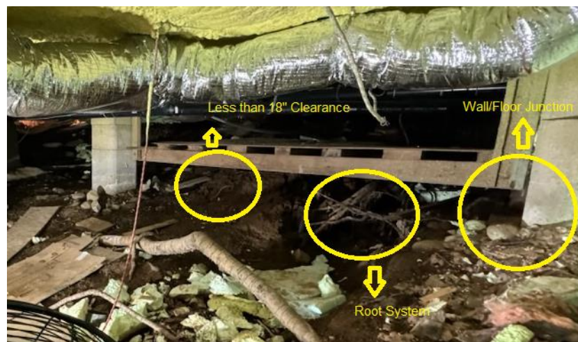
BEFORE – Clearance, protrusions and unreachable wall/floor junction
