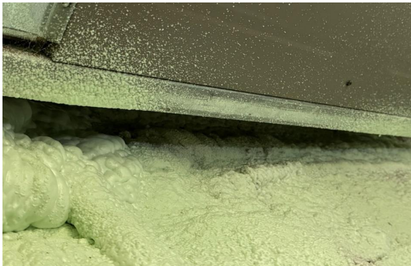
AFTER – complete seal with Boreal Elite ccSPF
