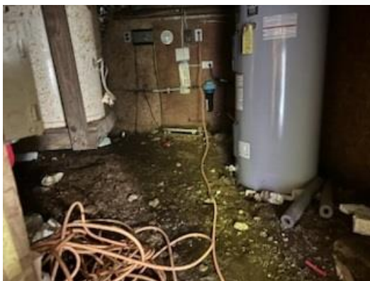
BEFORE - Clearance issues below water tanks
