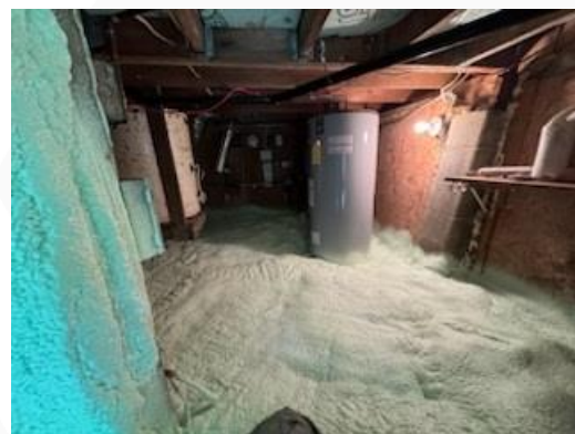
AFTER – Complete seal under appliances
