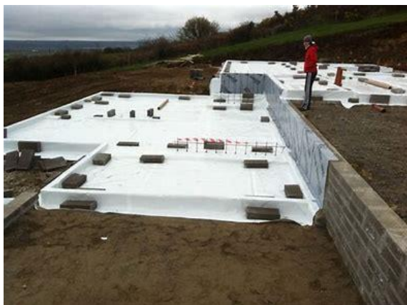
New construction membrane installation
