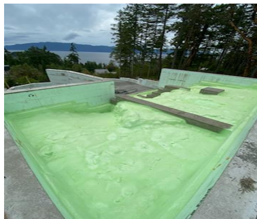
New construction Boreal Elite installation
