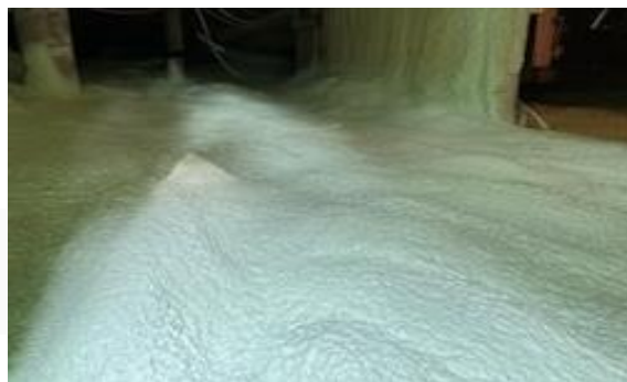
Before/After - ccSPF installed over rocks and root systems
