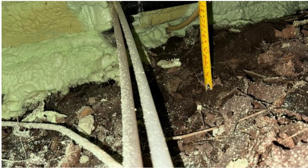
Areas of limited clearance – wall/floor junction less than eighteen inches
