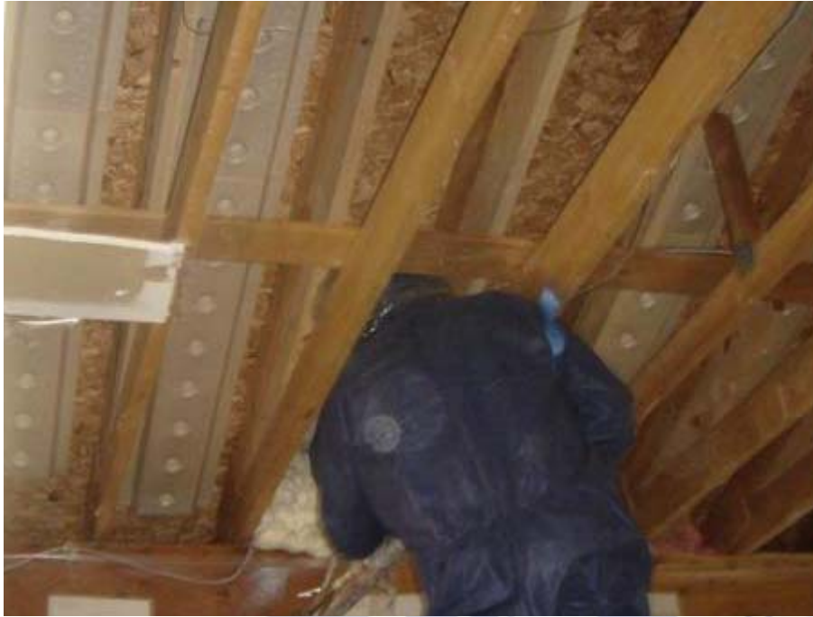
Figure 3 : Continuous baffles from the bottom to the top of the test assemblies
