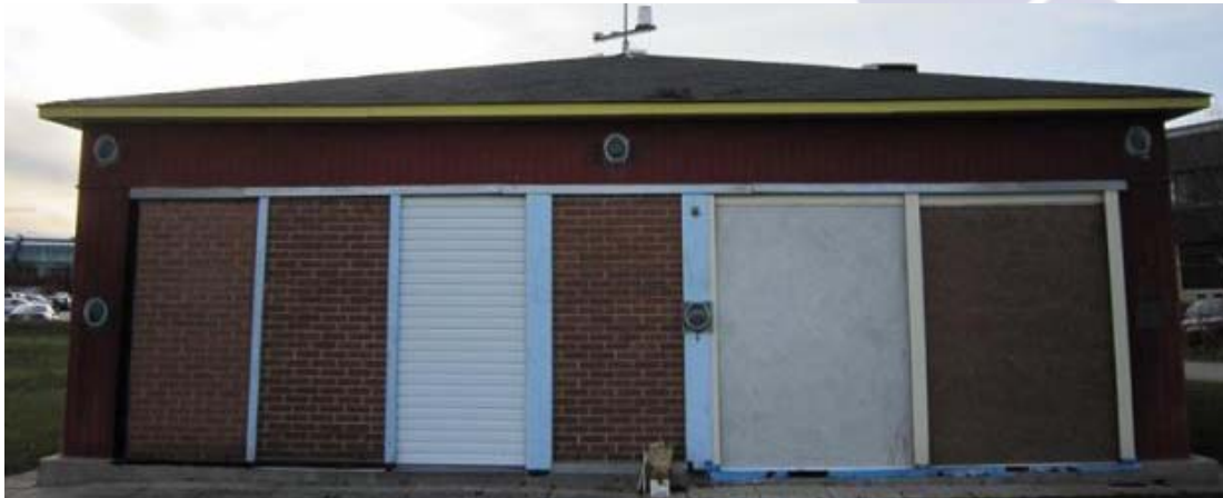
Figure 1 : Photo shows East orientation of test hut including hip roof
