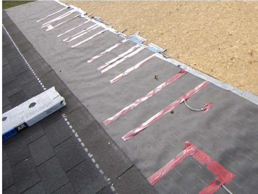
Figure 5 : Locations of wetting apparatus on the roof assemblies
