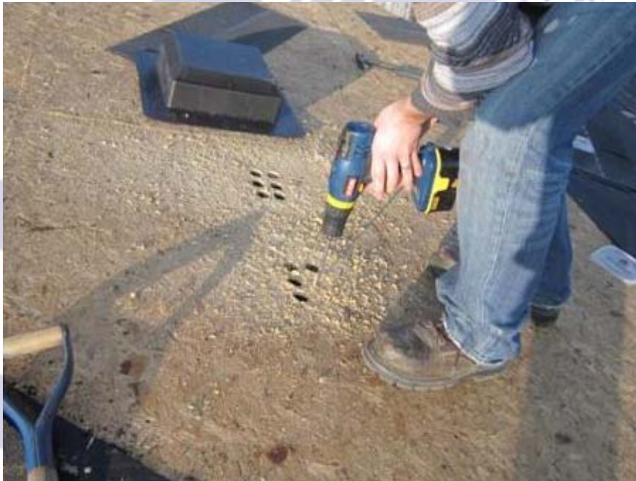
Figure 4 : Vent holes drilled in the roof sheathing and covered with vents
